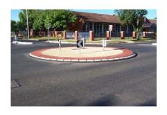
through the reduction of vehicle speeds and the nature of the vehicle conflict points within the intersection, the number and severity of accidents is reduced.
