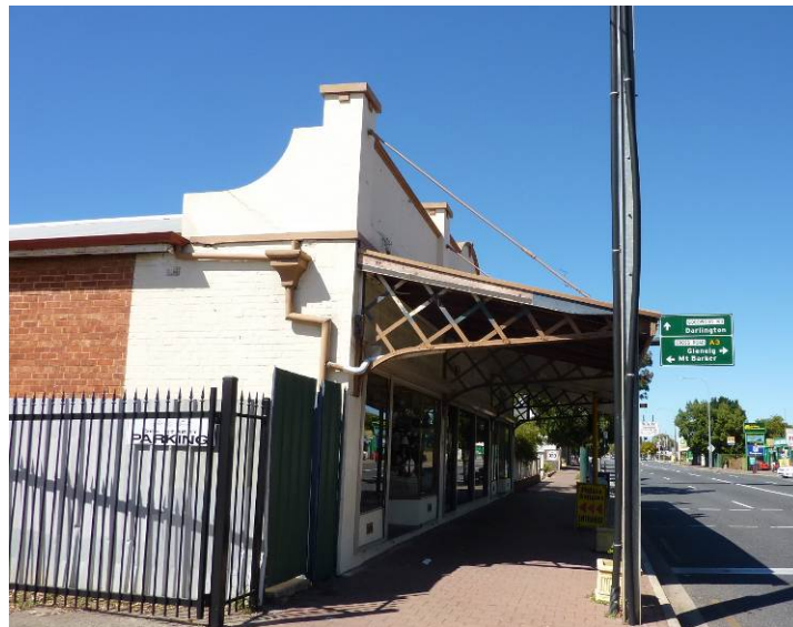
View south along Goodwood Road – showing lattice brackets
